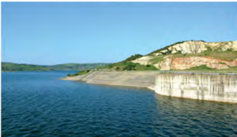
Views from Istanbul Sağırdere Dam
