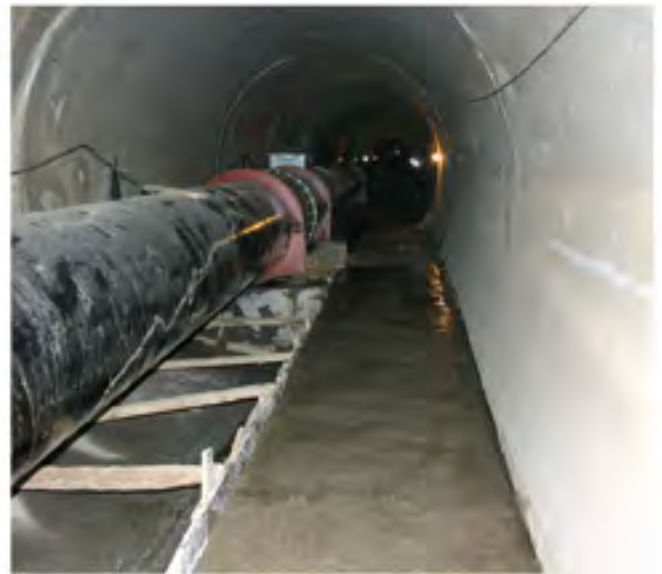
Views from the construction phases of Bingöl Gülbahar Dam
