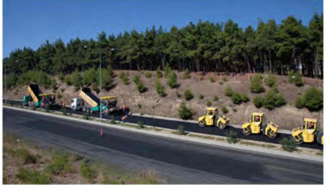
Road Construction Works at the Kıralı Disjunction-Tekirdağ Divided Road
