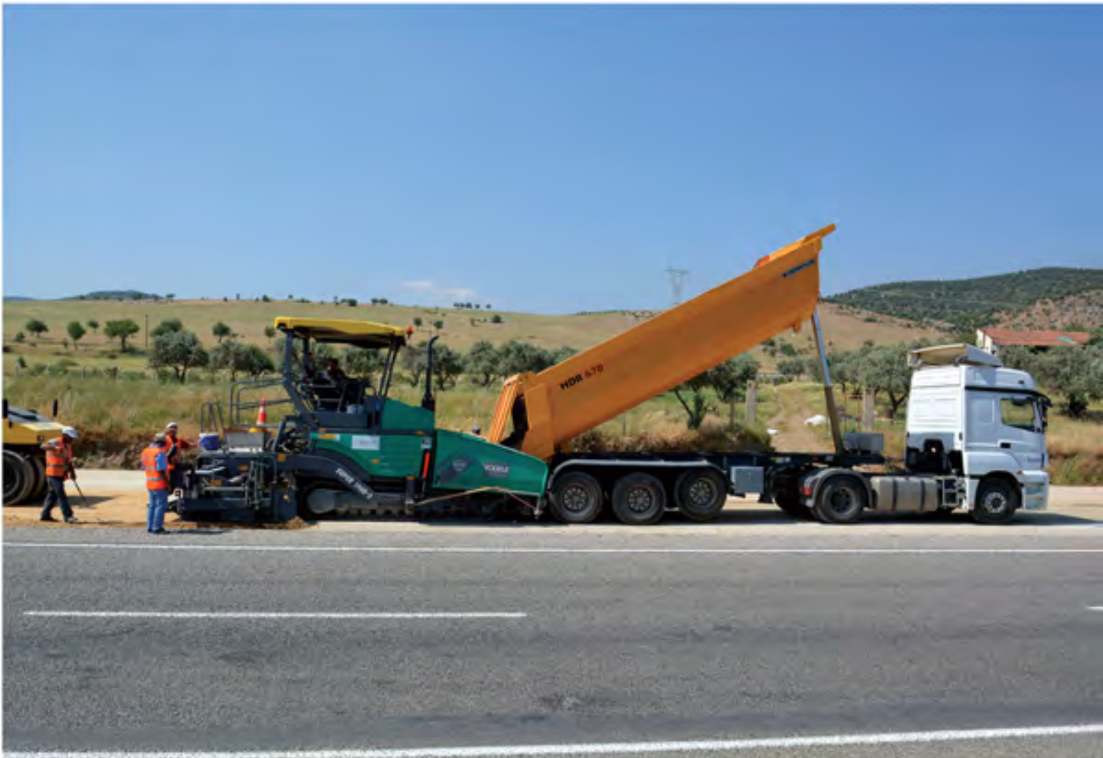
Divided Road Construction Works at Torbalı-Ödemiş-Kiraz Section
