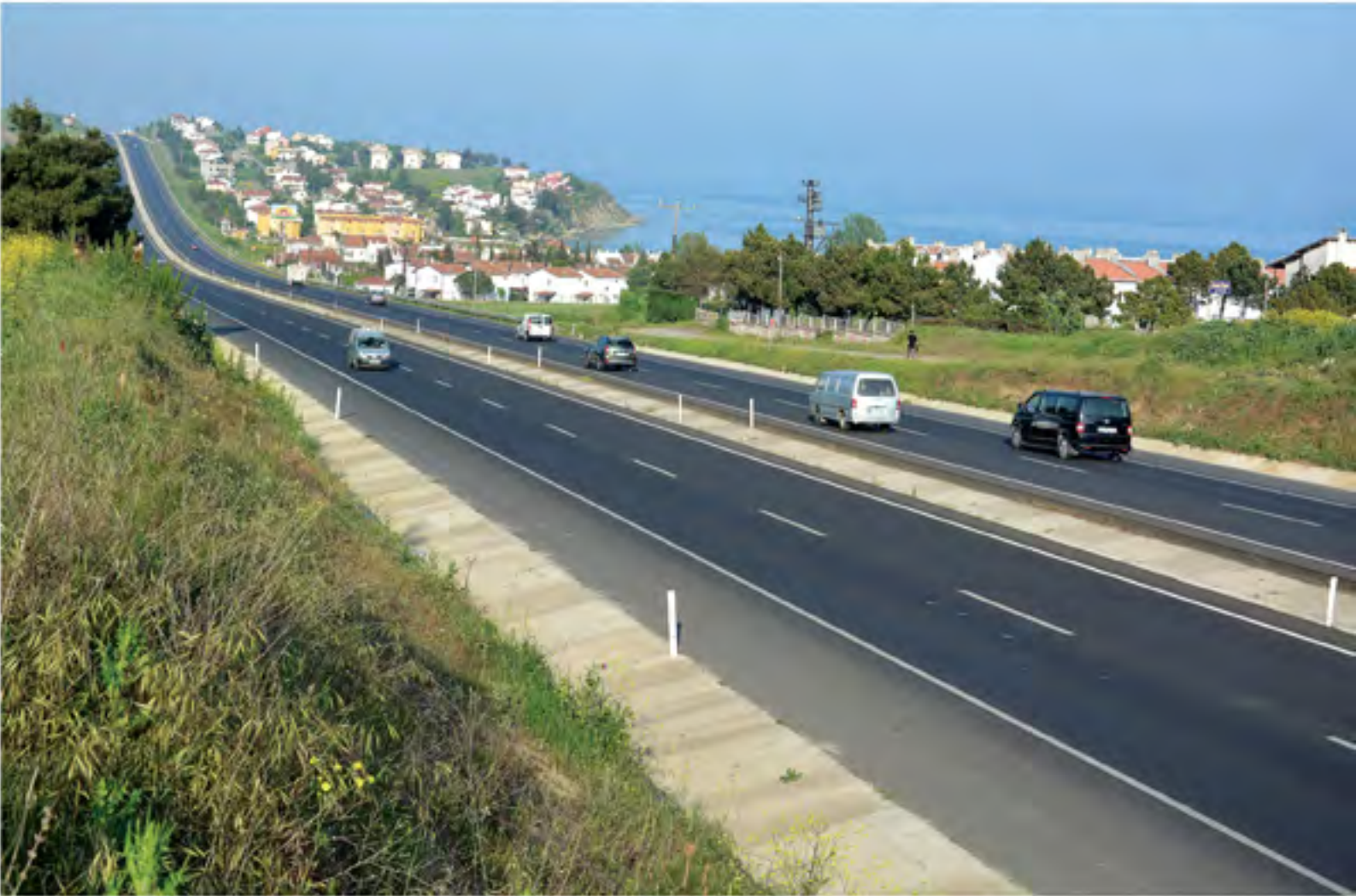
Various views from Kinalı Disjunction-Tekirdağ Divided Road
