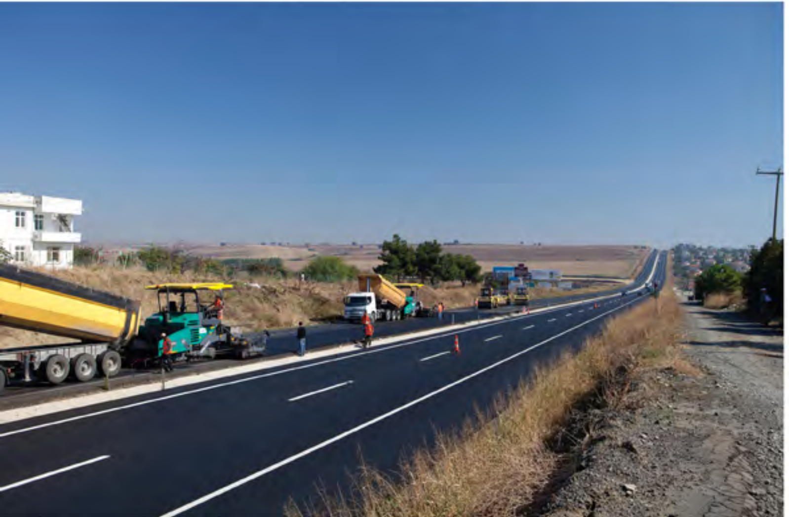
Road Construction Works at the Kınalı Disjunction-Tekirdağ Divided Road
