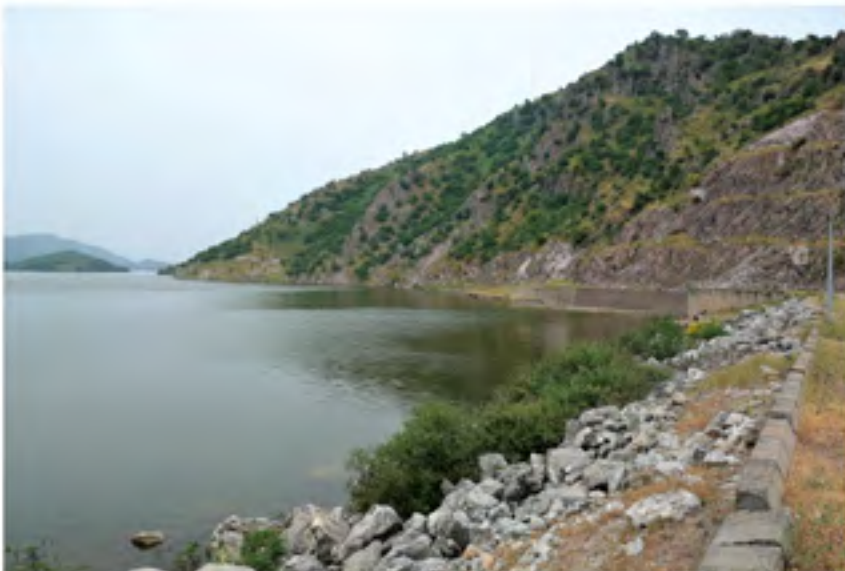
Views from Bergama Kestel Dam
