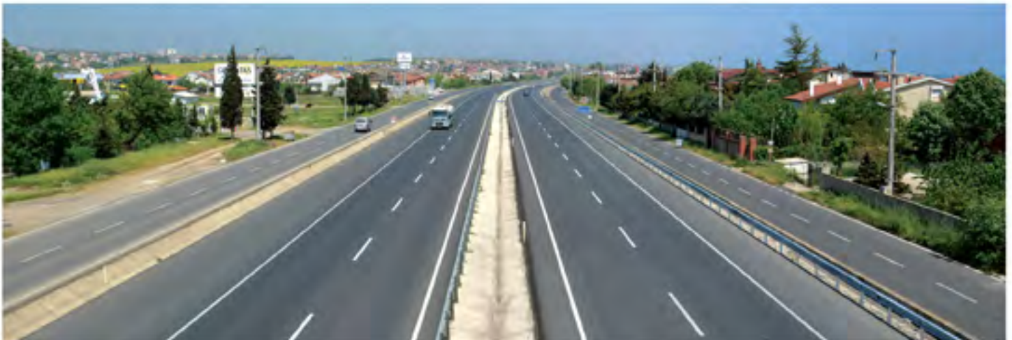
Various views from Kınalı Disjunction-Tekirdağ Divided Road
